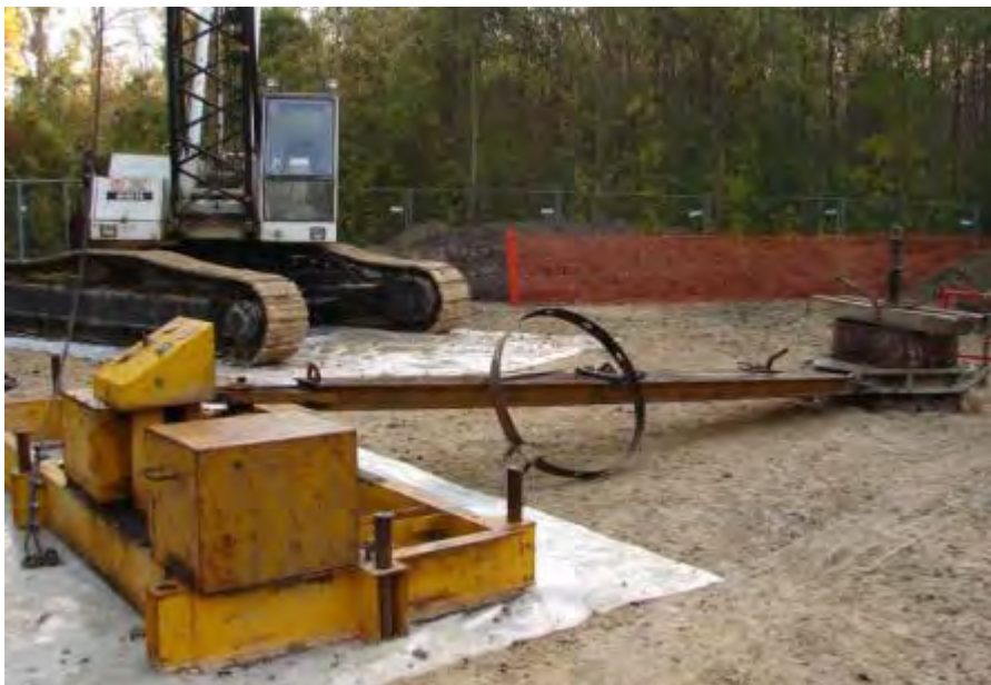
Figure 52. Grue de forage type BENOTO
