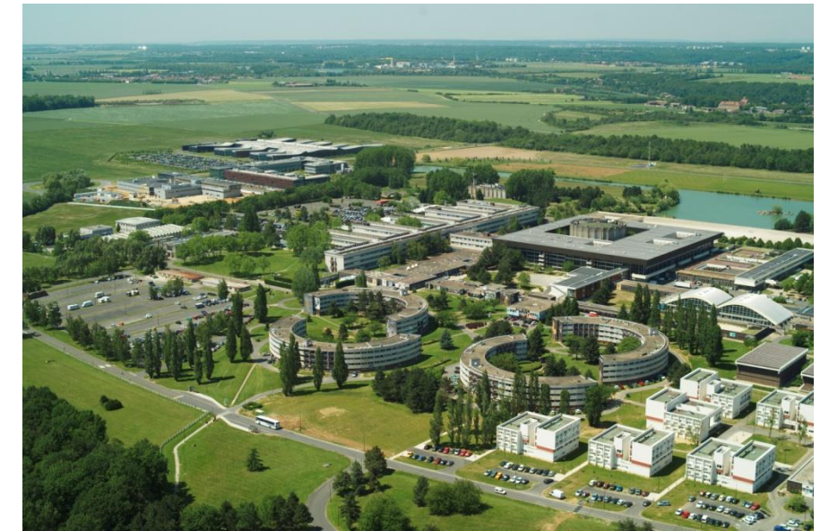
Figure 10. Le campus Polytechnique – site Ecole Polytechnique
